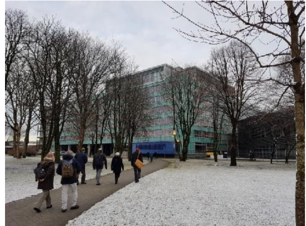
Figure 3: The building of the DB Operation Centre
