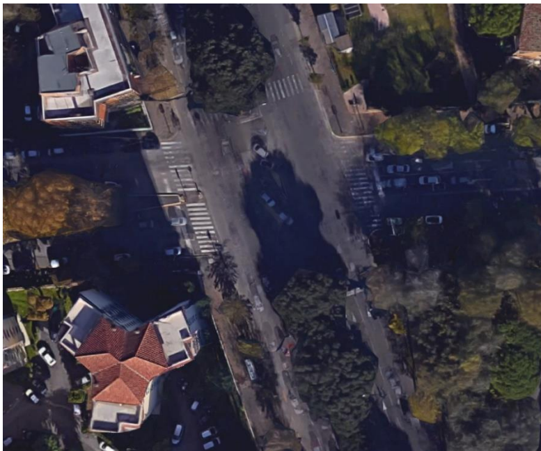
Figure 32: View of Intersection 11013
