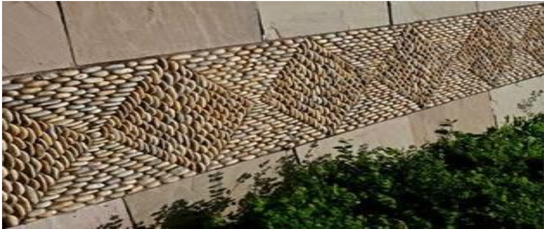
Fig. 4.5. Combination of cobblestone with stone slabs
