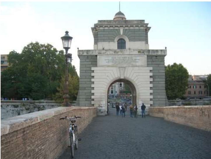
Ponte Milvio (start of Cycle Path from Ponte Milvio to Villa Ada)
