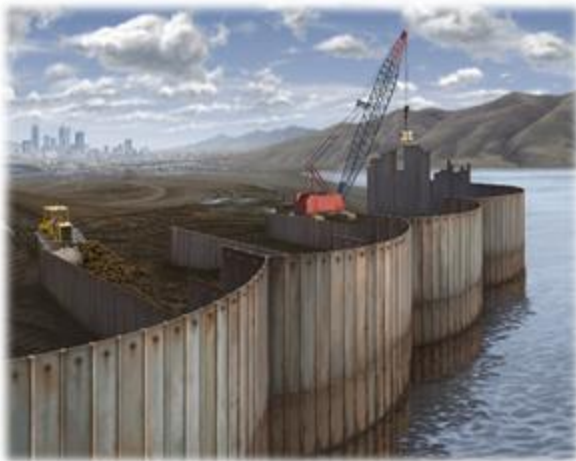
Figure 2-24. Sheet pile wall construction
