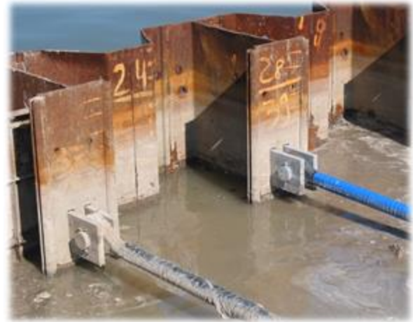
Figure 2-25. Anchored sheets of the wall
