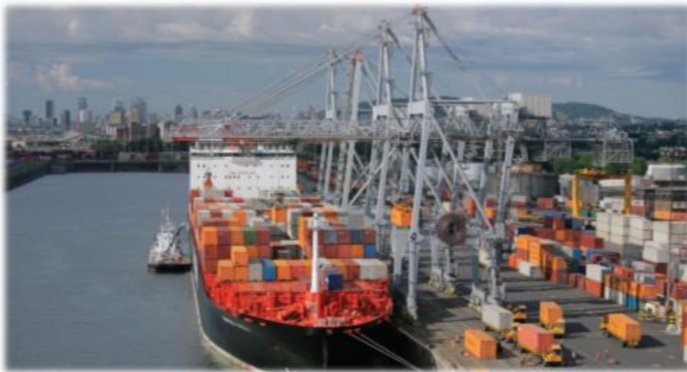
Figure 3-3. Panamax STS cranes, Racine Terminal, Port of Montreal, Canada (Liebherr, 2017)
