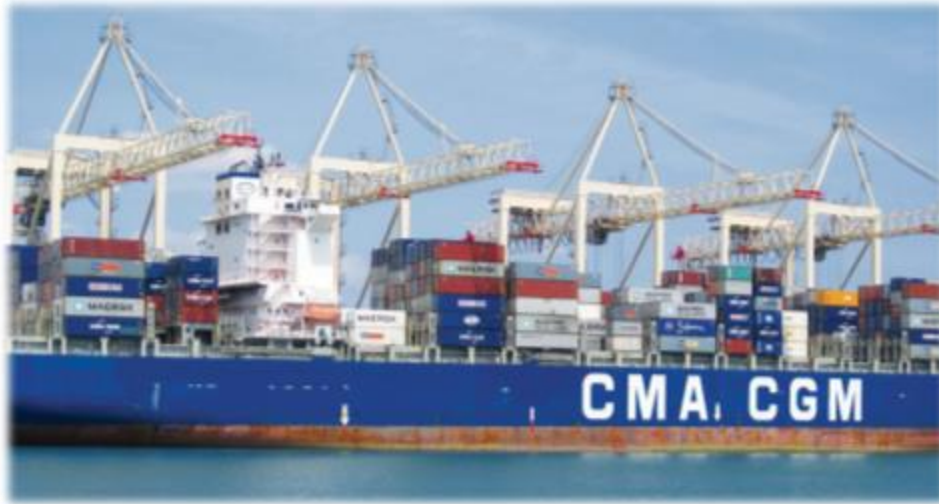
Figure 3-4. Post-Panamax ship to shore cranes, Koper, Slovenia (Liebherr, 2017)
