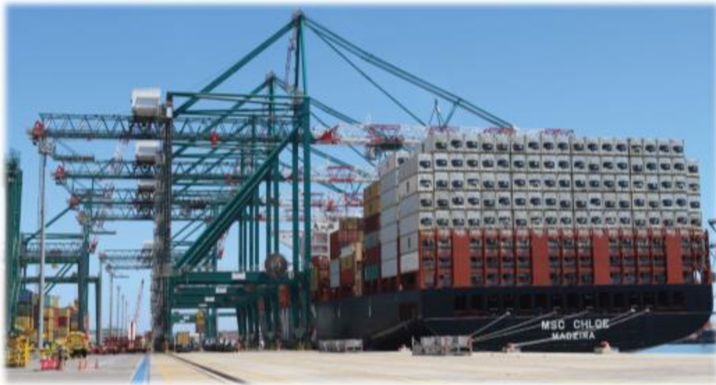
Figure 3-5. Super post Panamax STS cranes, Puerto Central, San Antonio, Chile (Liebherr 2017)
