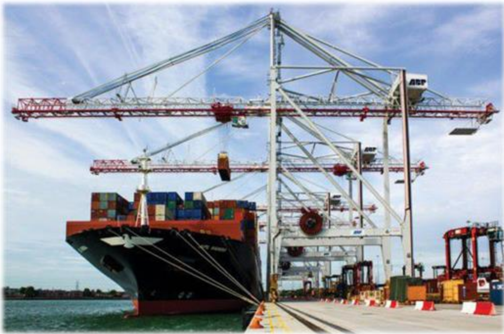
Figure 2-13. Gantry crane with thicker WSL (both legs are vertical)
