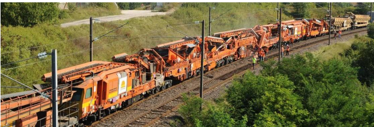
Picture 8 - ballast cleaning system for TGV lines, France
