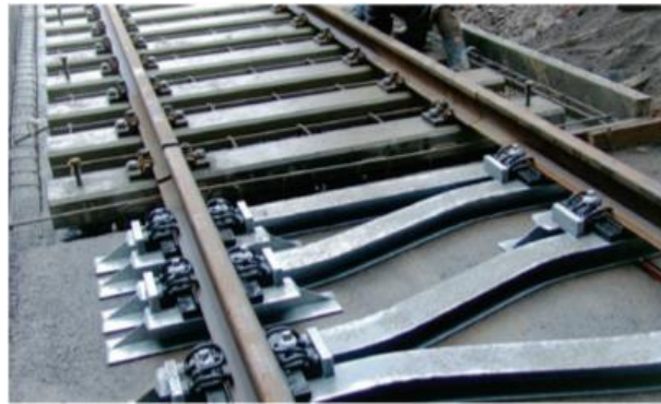
Picture 11 - SATO Y-shape sleepers
