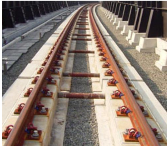
Picture 15 - Example of ladder track
