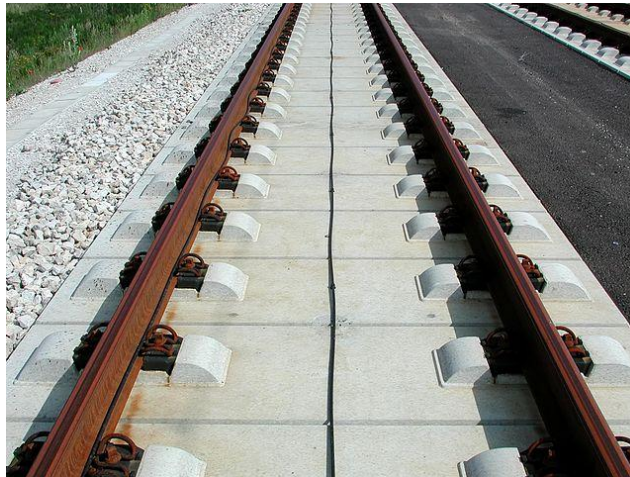
Picture 4 - FF Bögl Slab Track System
