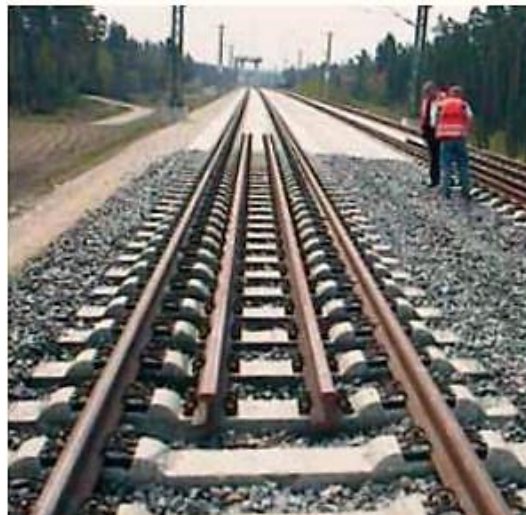
Picture 9 - Implementation of auxiliary rail (Rheda-system) [33]
