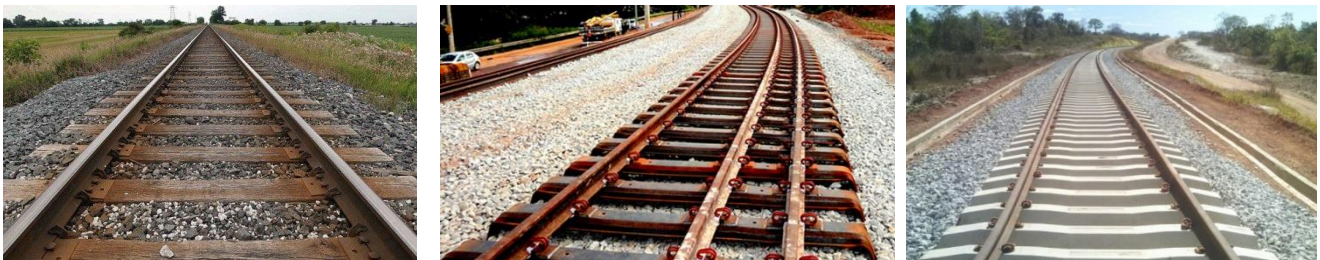
Picture 2 – From the left to the right: Wooden, steel, concrete sleepers
