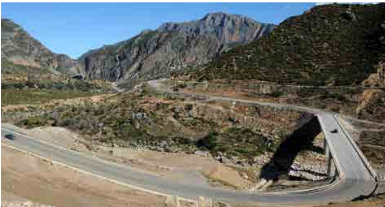
■ The road from Chefchaouen to Oued Laou, restored to improve infrastructure and create jobs in Morocco (AFP © EU/Neighbourhood Info Centre).
