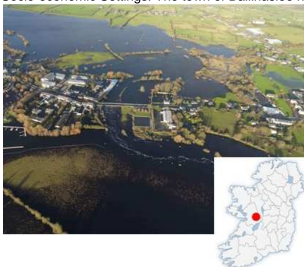
Figure 10 Aerial view of Ballinasloe when flooded in November 2009.
