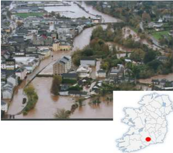
Figure 11 Aerial view of Clonmel in flood.
