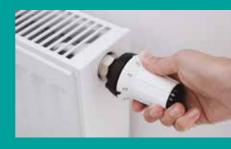
Equipping your radiators with a thermostatic valve allows you to save up to 20% of methane gas. In a year, you can save up to:
