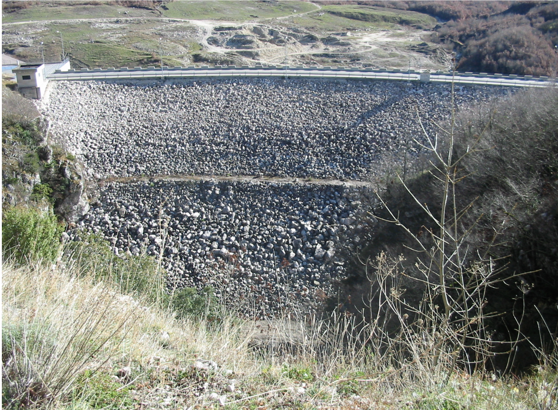
Arcichiaro, Italia BFRD – Bituminous Face Rockfill Dam (H=88 m)
