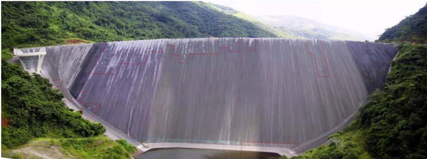
*Figure 3-Impervious facing at the end of the interruption period*
