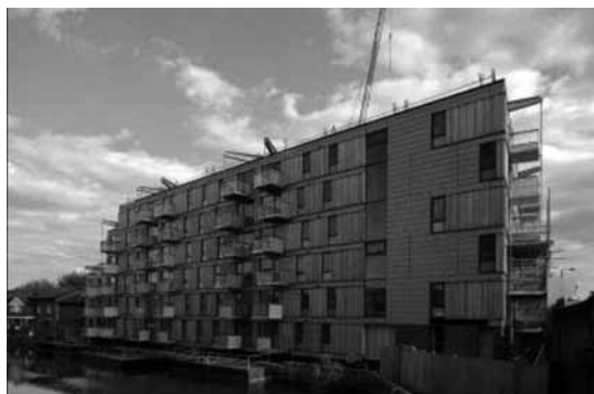
Adelaide Wharf, Hackney, Londra Adelaide Wharf, Hackney, Londres
